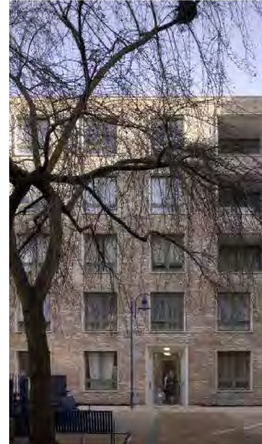
Peabody Housing, Whitechapel, London, Niall McLaughlin Architects. Nominated for the Stirling Prize 2015
