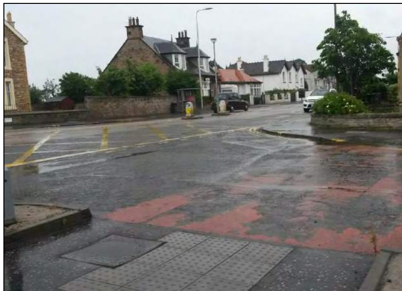
Dropped Kerb, tactile paving and pedestrian refuge at Brunstane Road South
