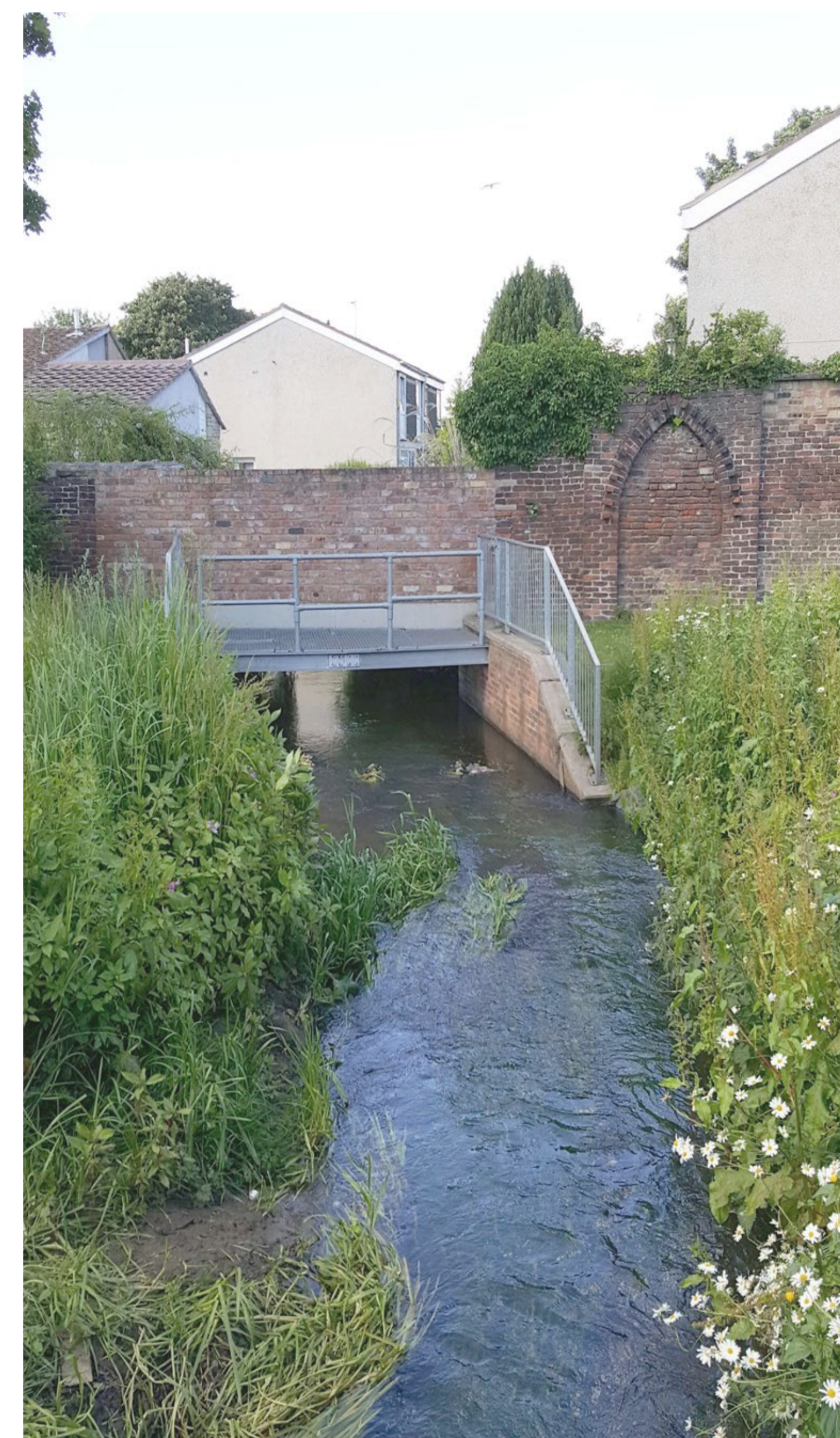
BRIDGE OVER FIGGATE BURN
