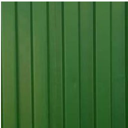
Painted metal external walls (Moss Green - RAL6005) (cabins)
