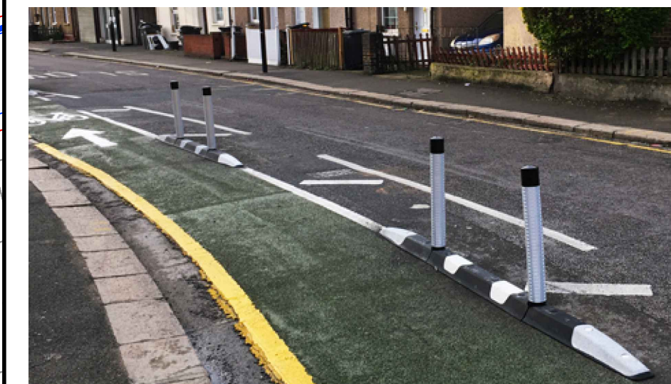
Fig 1. ORCA WAND - TO PROVIDE TRAFFIC SEGREGATION. PRODUCT 2.5m IN LENGTH & ARE BOLTED INTO CARRIAGEWAY WITH 5m GAP.
