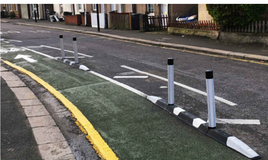
Fig 1. ORCA WAND - TO PROVIDE TRAFFIC SEGREGATION. PRODUCT 2.5m IN LENGTH & ARE BOLTED INTO CARRIAGEWAY WITH 5m GAP.
