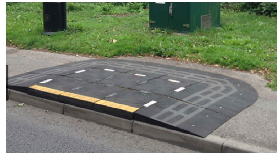
Fig 2. REDIWELD BUS PAD (OR SIMILAR)- RETAIN BUS STOPS WHERE NO LAYBY PROVIDED.
