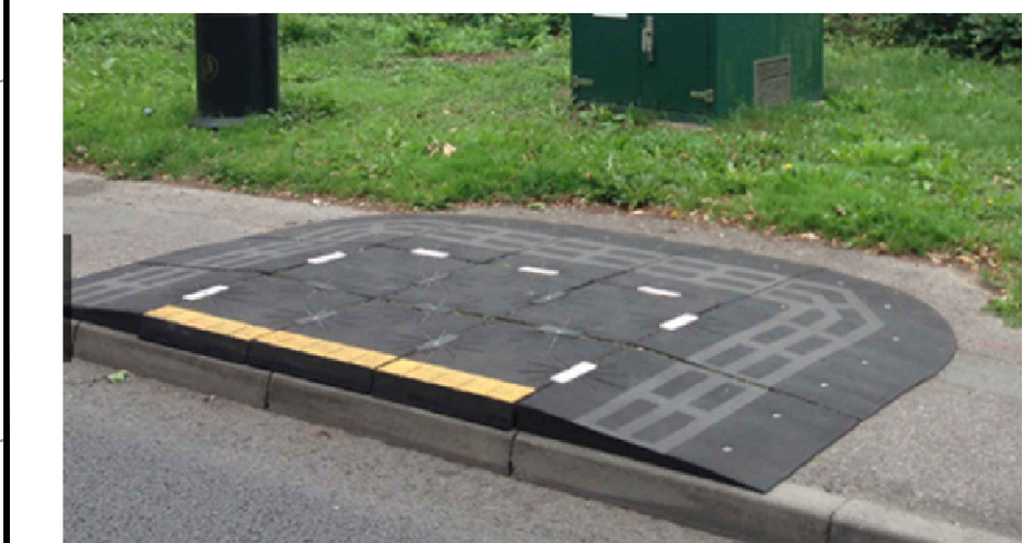
Fig 2. REDIWELD BUS PAD (OR SIMILAR)- RETAIN BUS STOPS WHERE NO LAYBY PROVIDED.
