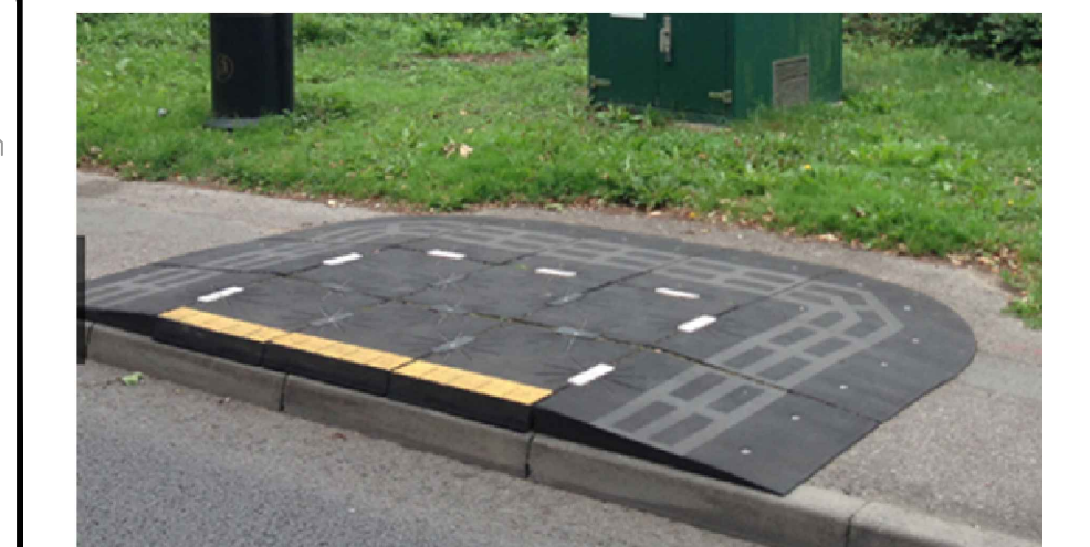
Fig 2. REDIWELD BUS PAD (OR SIMILAR)- RETAIN BUS STOPS WHERE NO LAYBY PROVIDED.
