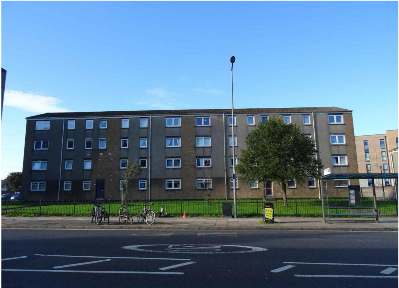
Figure 1 - Site Photograph. Aspect of street furniture and trees
