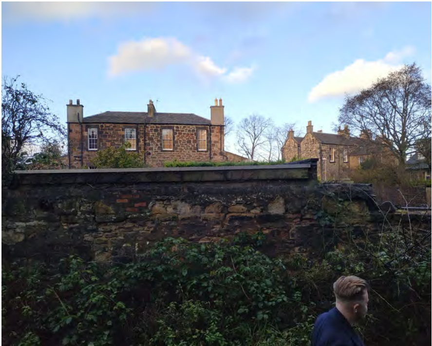
03 Any replacement of the wall would require the partial demolition of the lock ups with retaining work required.
