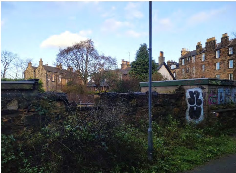
02 Rear Boundary wall backing on to Christians Public Pathway, is in great need of replacement and has deteriorated badly and is close to the point of failure.
