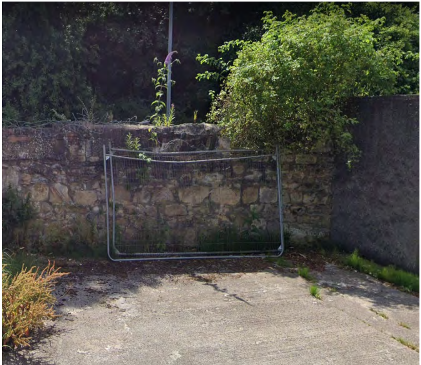
04 Rear Boundary wall backing on to Christians Public Pathway, is in great need of replacement and has deteriorated badly and is close to the point of failure.
