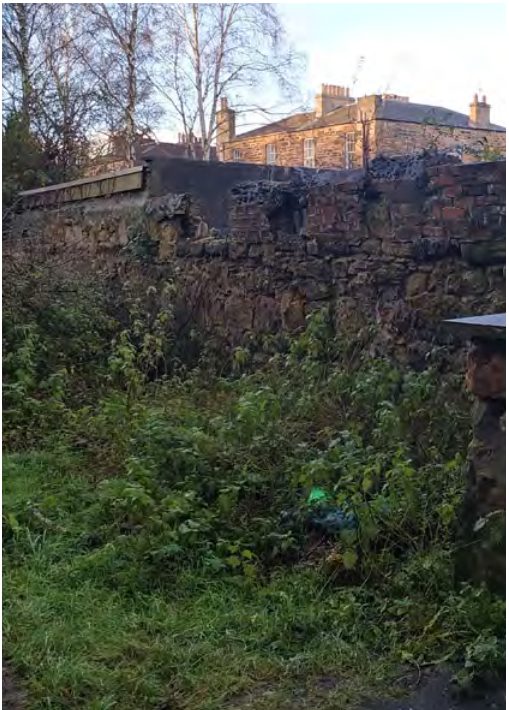
05 Poor areas of brick & mortar have been used to built the wall back up however parts of this have already broke away, crumbling away.
