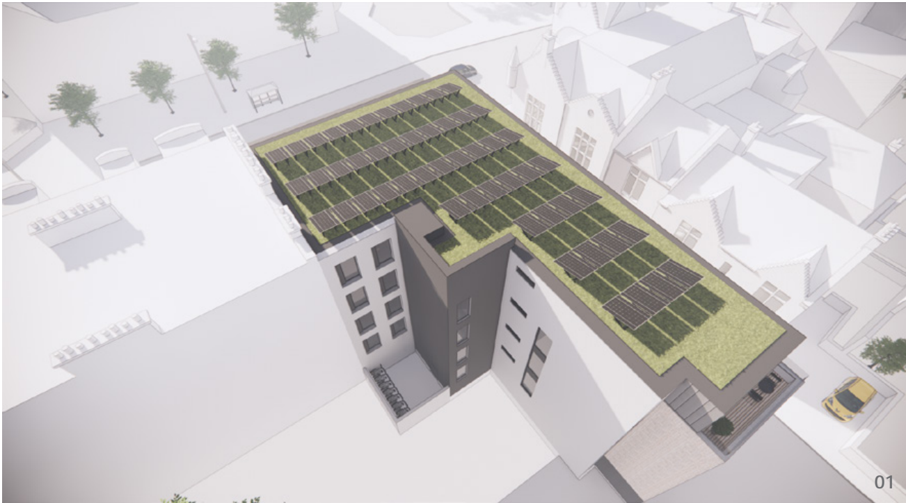
01 Solar Panel Placement shown to flat roof. Location of panels have been setback from the street edges of Portobello High Street & Beach Lane.
